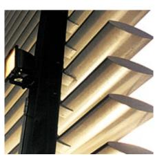
▲ Birdsmouth brackets. Horizontally mounted c|sairfoil AF270 blades are shown from behind the facade of a building. Birdsmouth brackets had been fixed onto vertical support segments at specified distances and c|sairfoil blades were then simply slotted into the brackets and fixed with screws or rivets. Birdsmouth brackets allow for speedy onsite installations and have the additional advantage of being virtually invisible when seen from the front.
