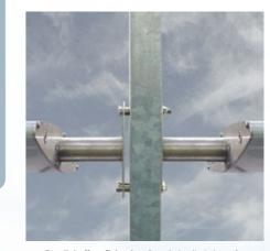
▲ Parallel offset fixing bracket. A detailed view of an 270F blade onto a vertical support segment is illustrated in a wide variety of angles cater for an unlimited range of design possibilities and adapt to virtually any project
