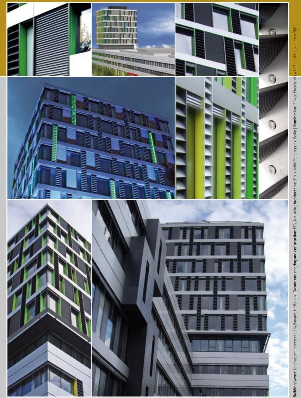
Project Landratsamt Heilbronn: Colour LEDs integrated into the embrasures of windows illuminate at night horizontally arranged noiseabsorbing CS Airfoil AF320 LB solar shading blades to make the illuminated building also at night a focal point of attention.
