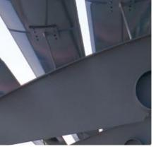
Custom blade supports. The custom blade supports shown have been specifically designed for cantilevered projections of Audi showrooms. c|sairfoil AF270 blades are fixed onto vertical custom-made supports, attached to horizontal support seaments. The lightweight but extremely robust structure of clsairfoil blades allow for the design of any imaginable support, fixture, suspension or attachment. This results in an extremely versatile, architectural design
